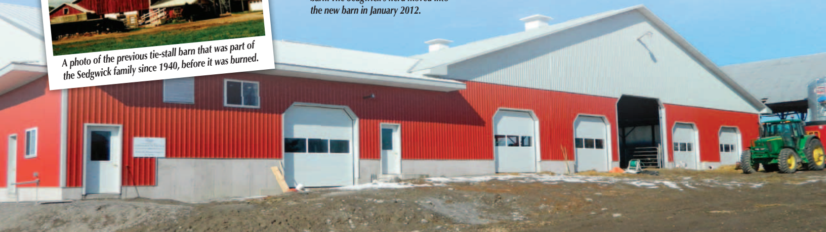
A state-of-the-art free-stall barn now stands in place of the existing tie-stall barn. The Sedgwick's herd moved into the new barn in January 2012.
