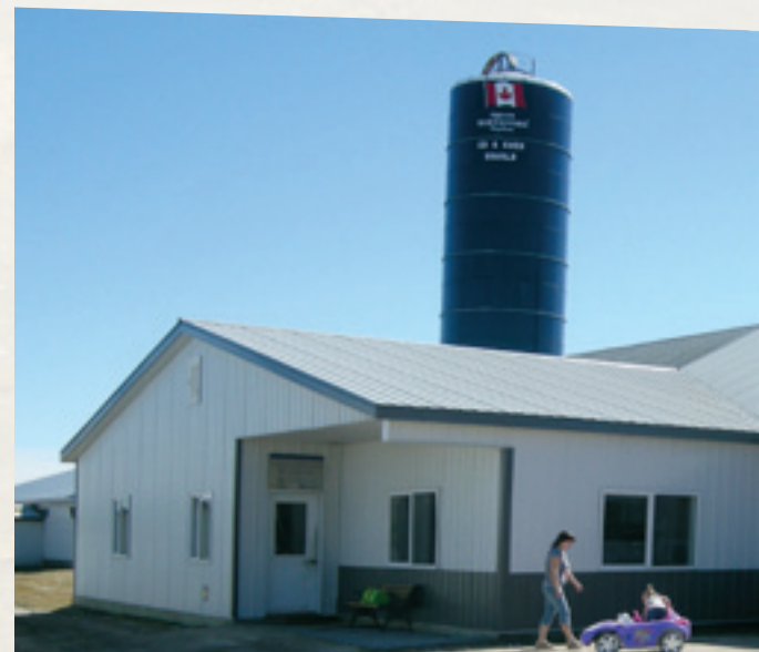
Cottonwood's second free-stall barn was constructed in 1975.
